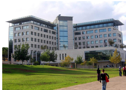
Technion Computer Science Faculty Building
